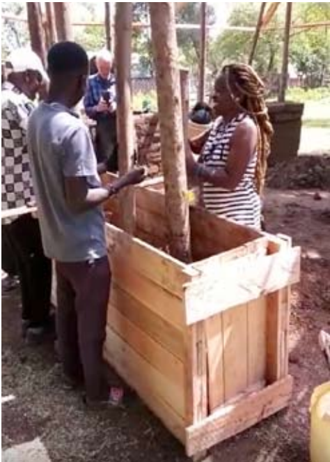
(top left) The wooden box was used for ramming the walls whereby soil was put inside it and rammed down. (top middle) These people were building the walls with clay bricks. (top right) The person on top of the roof was making the roof with grass. (middle left) Dancan working with friends from France in the garden planting seeds in the keyhole garden with vegetables, as shown below it. (middle right) The Adobe brick house finished with only the four windows and the floor to be fitted. (bottom left) Dancan teaching a microbiotic way of living and permaculture in a local church.
