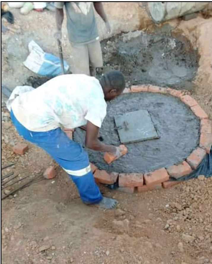
(top left) Bigboy (in yellow shorts) with the workers in the background getting the ground ready for the well. (top right) Assessing progress after the hole was dug. (bottom left) The Madzibaba brothers are laying bricks around the well, and (bottom right) – voilà – the finished well!
