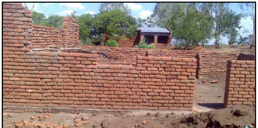
Printernet Project building under construction.
