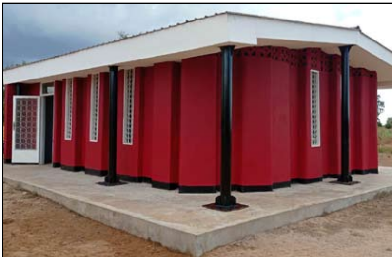
The new 3D-printed school in Salima, made of concrete placed layer by layer through a computer-controlled nozzle, in central Malawi, June 18, 2021.
