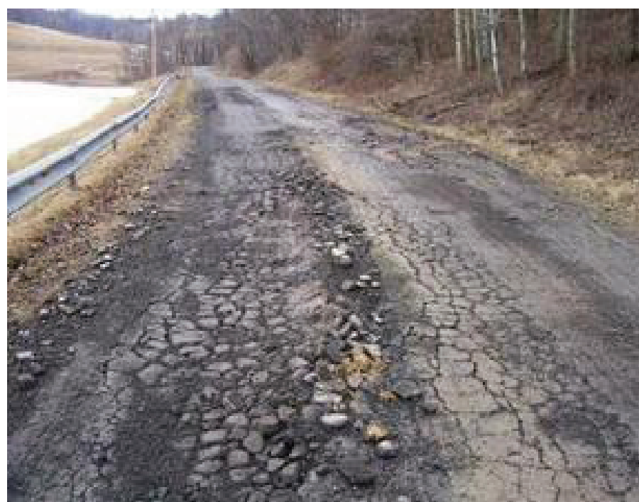
(left) Anthony Crane blocks road for hours on Route 89 on December 23, 2010. Photo from Wetzel County Action Group. (right) Road in Wetzel County damaged by gas drilling trucks. Photo by Paul Sands
