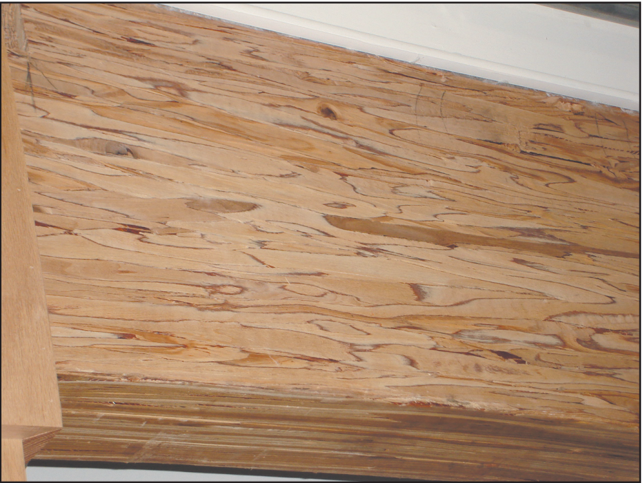
This sturdy beam was made from recycled plywood veneers. Serving the Northern Virginia, D.C. and Maryland regions, the Green Building Institute is a non-profit organization which educates the public as well as building and design professionals about sustainable building practices and technologies. Photo by Iona
