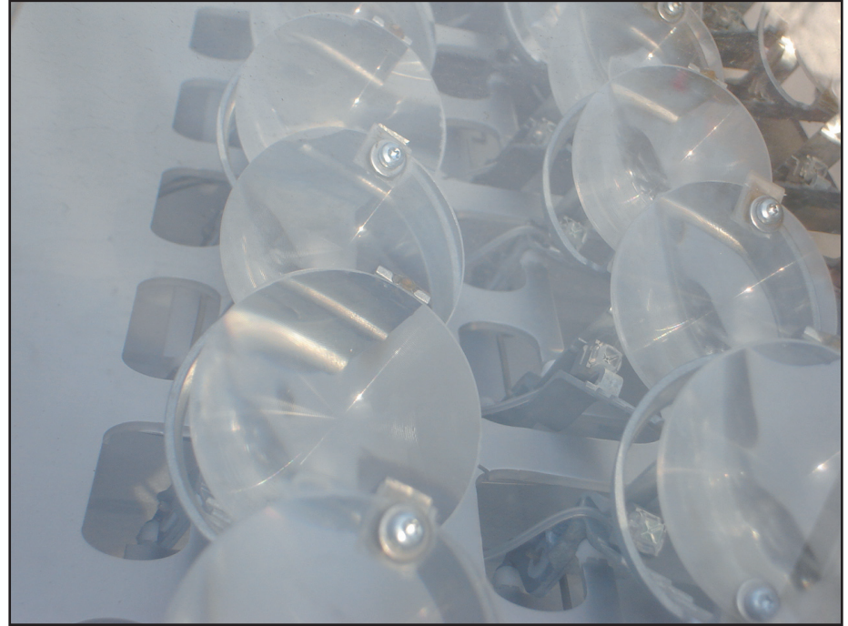
Small solar collectors move with the sun. This is one of the latest designs in capturing the sun's light and transferring it to the inside of the building through fiber optics. Green building is the practice of increasing the efficiency with which buildings use and harvest energy, water and materials. Photo by Iona
