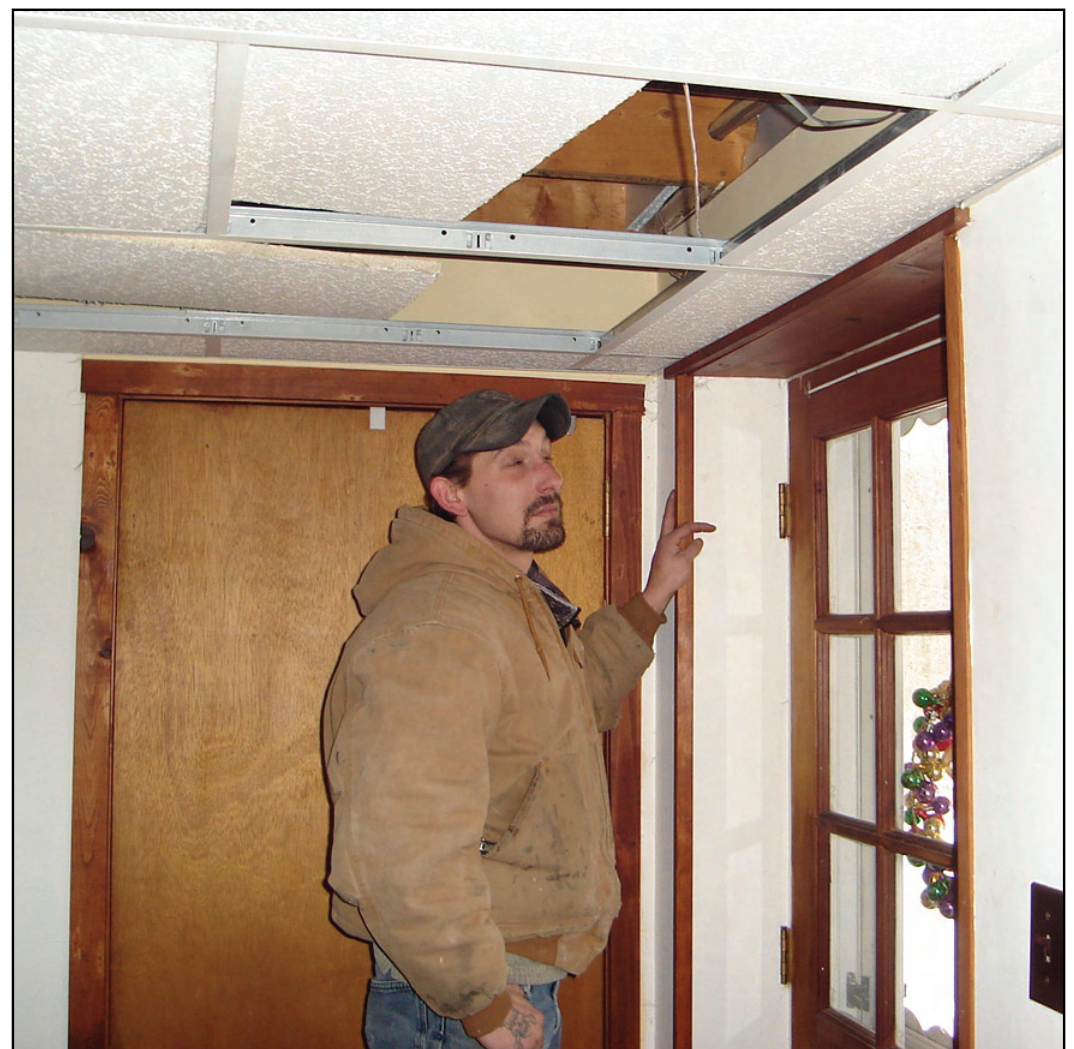
Rob Smith put styrofoam sheets all along the perimeter of the basement above the cinder block and caulked them to tighten up the ground level.
