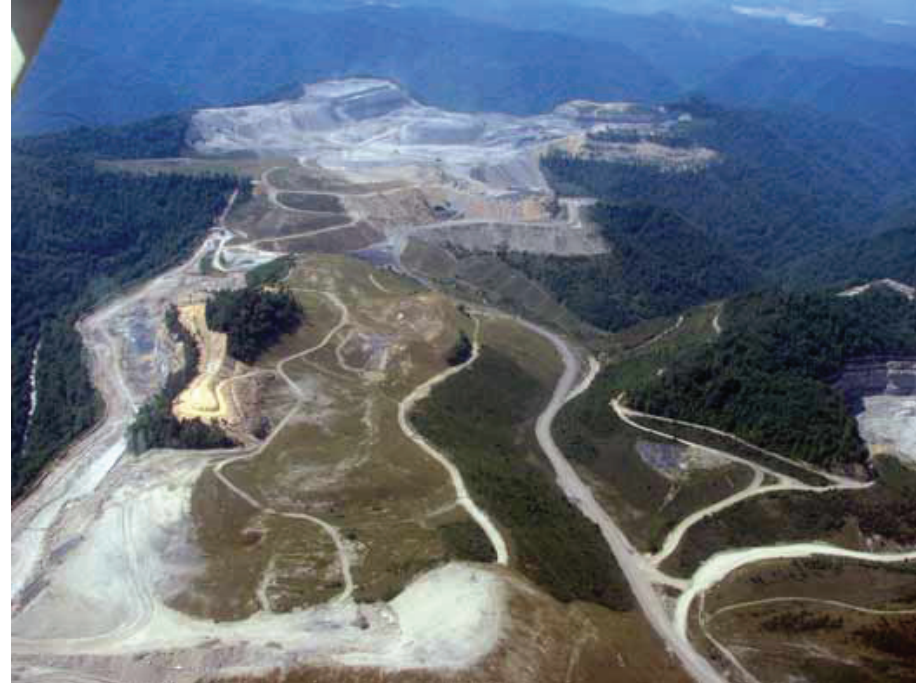
Photo #2: Sludge Pond. These artificial ponds are filled with a toxic semi-liquid sludge that is a safety worry to all that know that these impoundments have been known to leak and break, especially during times of heavy rain. West Virginians remember the 2000 Kentucky impoundment failure "... what federal officials called the worst environmental disaster in southeast U.S. history ... ." (www.loe.org). Residents recall numerous floods of '03 and '04, the May '02 flood in McDowell Co., the Massey Valley Fill Disaster in '02 and the 1972 Buffalo Creek disaster that killed 127 people and injured over 1,000 in which hundreds of homes were lost, not to mention the environmental impact. Families near MTR sites continue to create lists of contaminants found in their drinking water: arsenic, manganese, lead, barium, selenium, aluminum (www.pbs.org), and the list continues to grow. "It's estimated that there is over one hundred billion gallons [of coal sludge/slurry] amassed in active WV impoundments (Moyers'Journal www.pbs.org)." That's 110,000,000,000 gallons!
