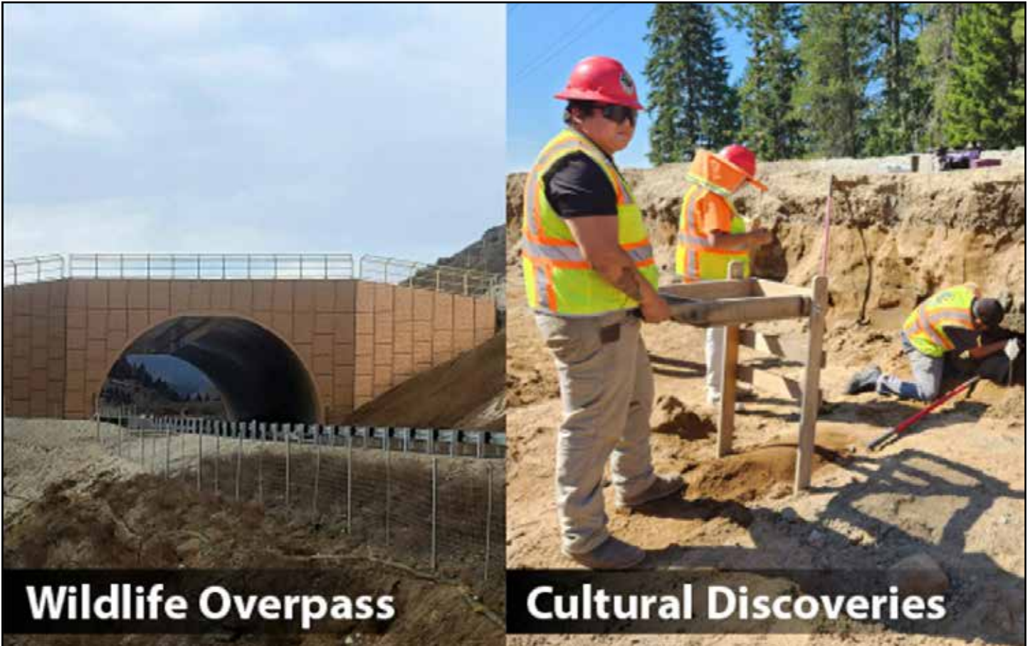
U.S.-95 McArthur Lake Bridge construction.
